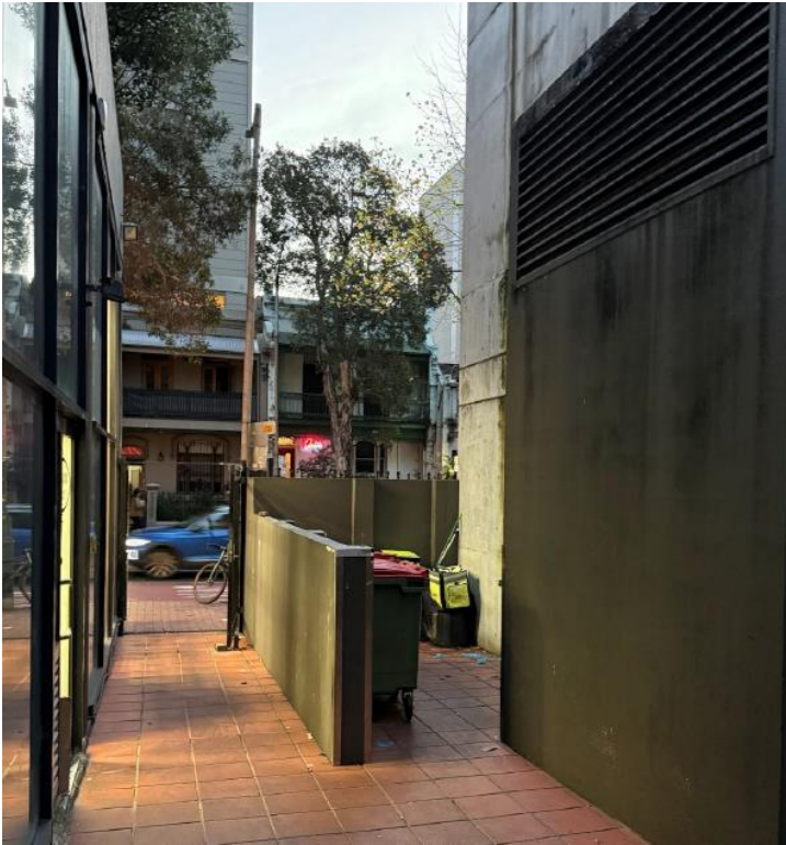
Figure 5: Shared waste storage area at northern edge of tenancy, looking west towards Elizabeth Street
