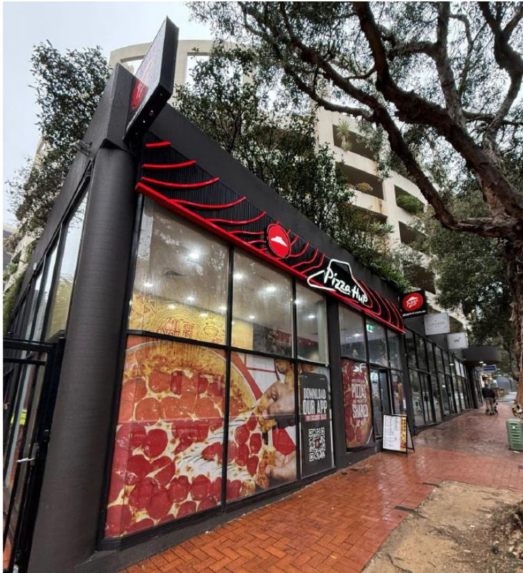
Figure 3: Site viewed from Elizabeth Street footpath
